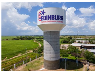
1-Million Gallon Water Tower Project
